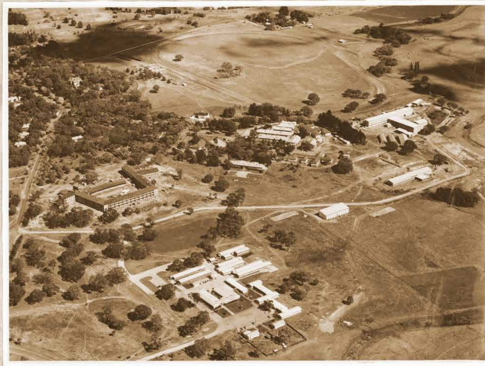
Administration and temporary buildings of the John Curtin School of Medical Research.
