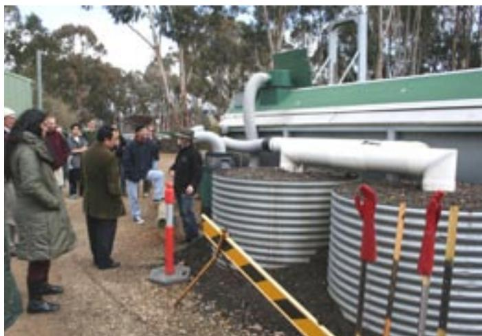
As decomposition occurs a pungent ammonia - laced odour is released. ANUgreen devised its own bio-filter, with assistance from R5 Solutions (NZ), consisting of soil filled tanks (seen here) to reduce the smell. So far it seems to have worked but the real test may come in summer.
