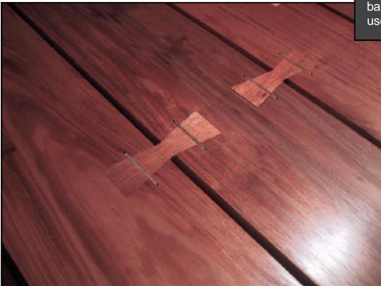
▲▲ The butterfly joints are held in place with twine recessed into the wood.
