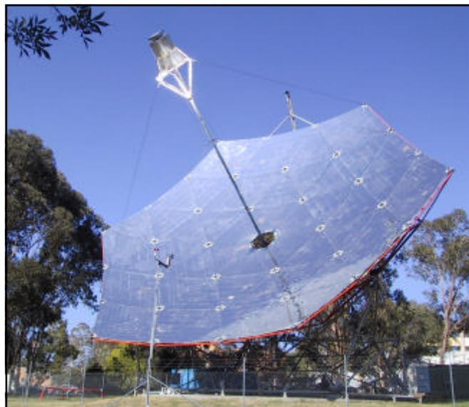
▲▲ By simply replacing the glass on the mirrors of the Big Dish with low-iron glass you can harvest an additional 5% of the sunlight.
